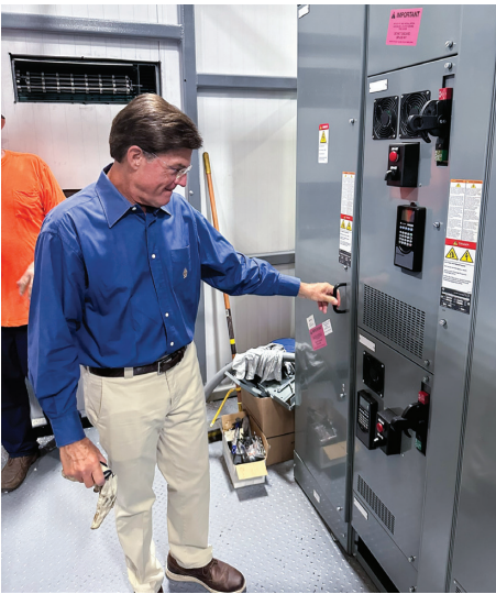
Founder and CEO Tim Tilley inspects one of the mechanical rooms being constructed by Envirosep.
