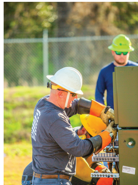
Channing Matthews and his Santee Electric crew change out a padmount transformer during the S.C. Lineworkers Rodeo.
